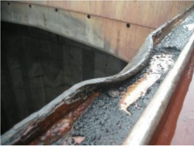
Figure 2: Damaged cargo hatch sill
