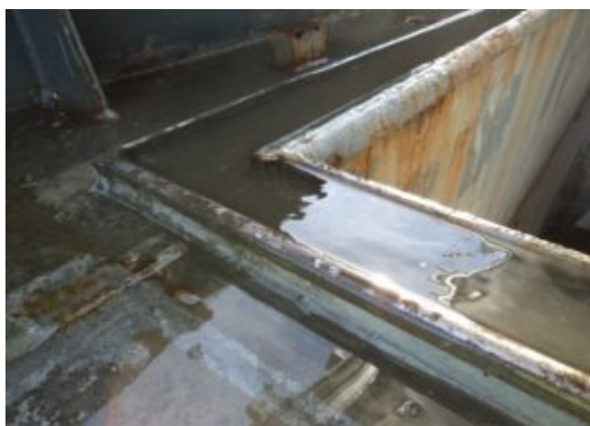
Figure 3: Overflowing drainage channels
