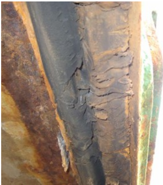
Figure 5: Hardened indented rubber seals
