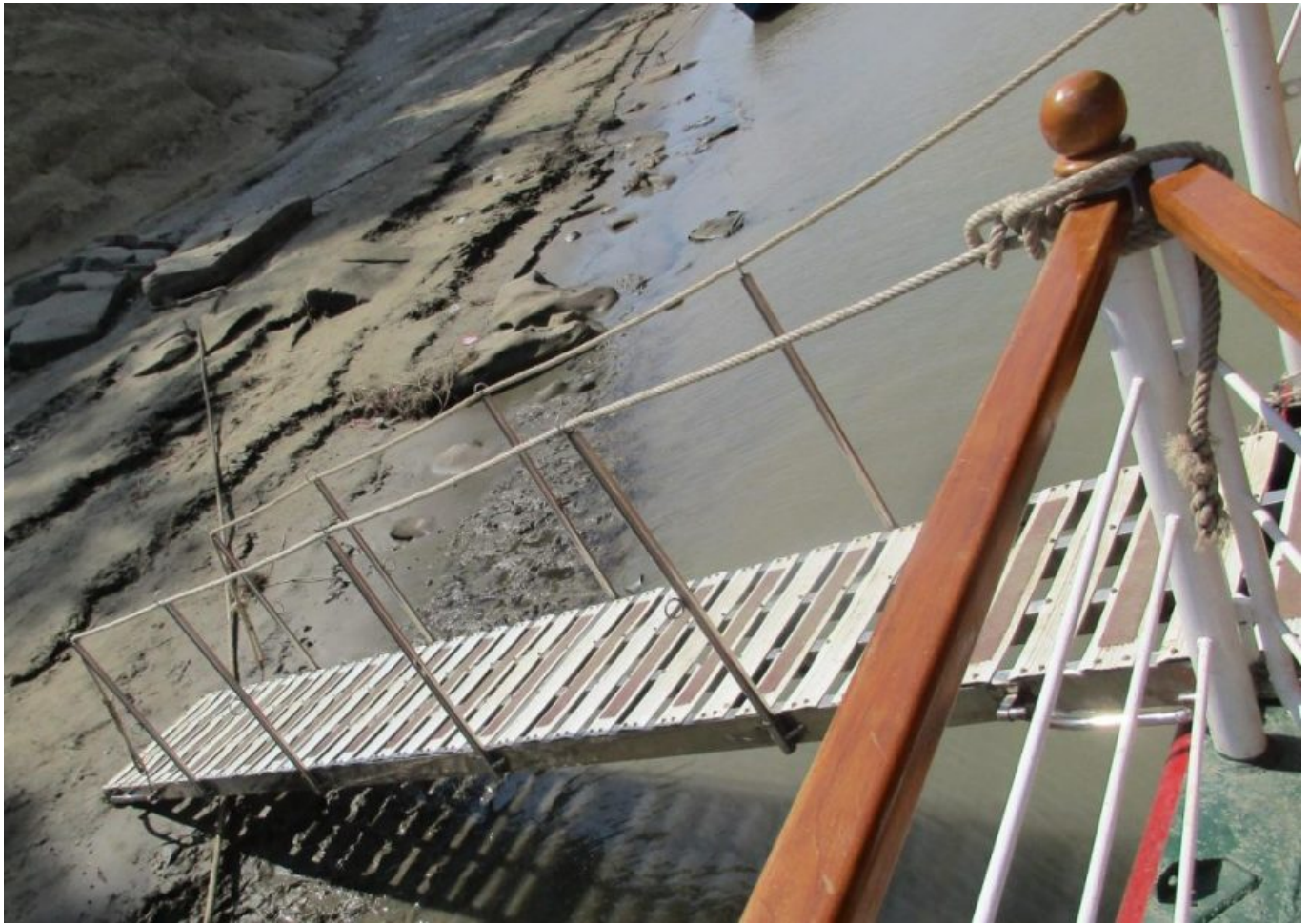
Example C: Gangway has not been manufactured by recognised national or international standards, is not properly secured, has no side screens or handrails provided and is not well lit.
